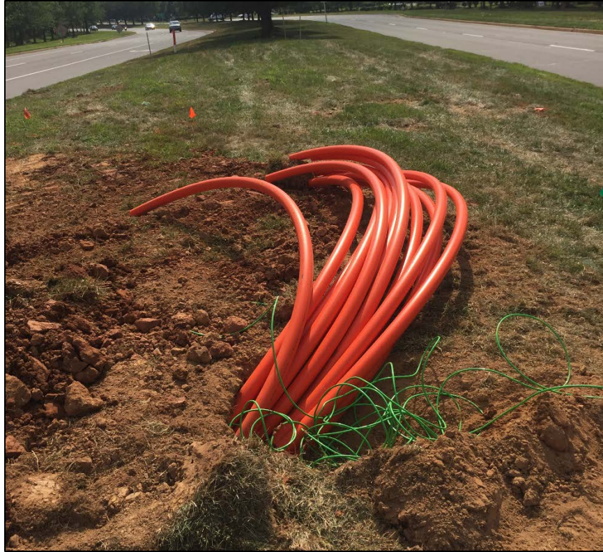
Figure 3: HDD Installation of HDPE Conduit
