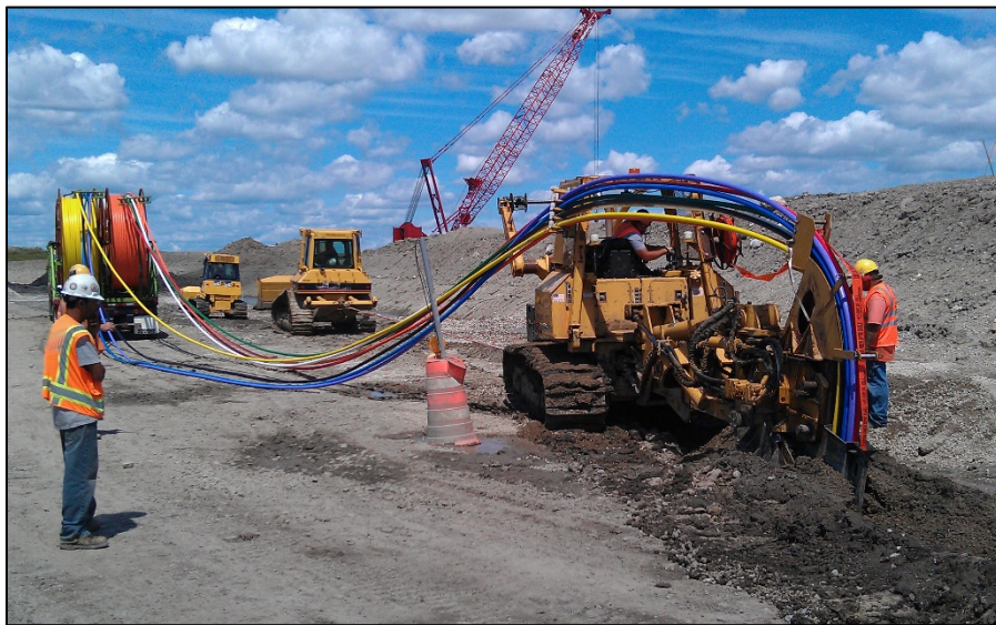
Figure 2: Plowing Installation of HDPE Conduit
